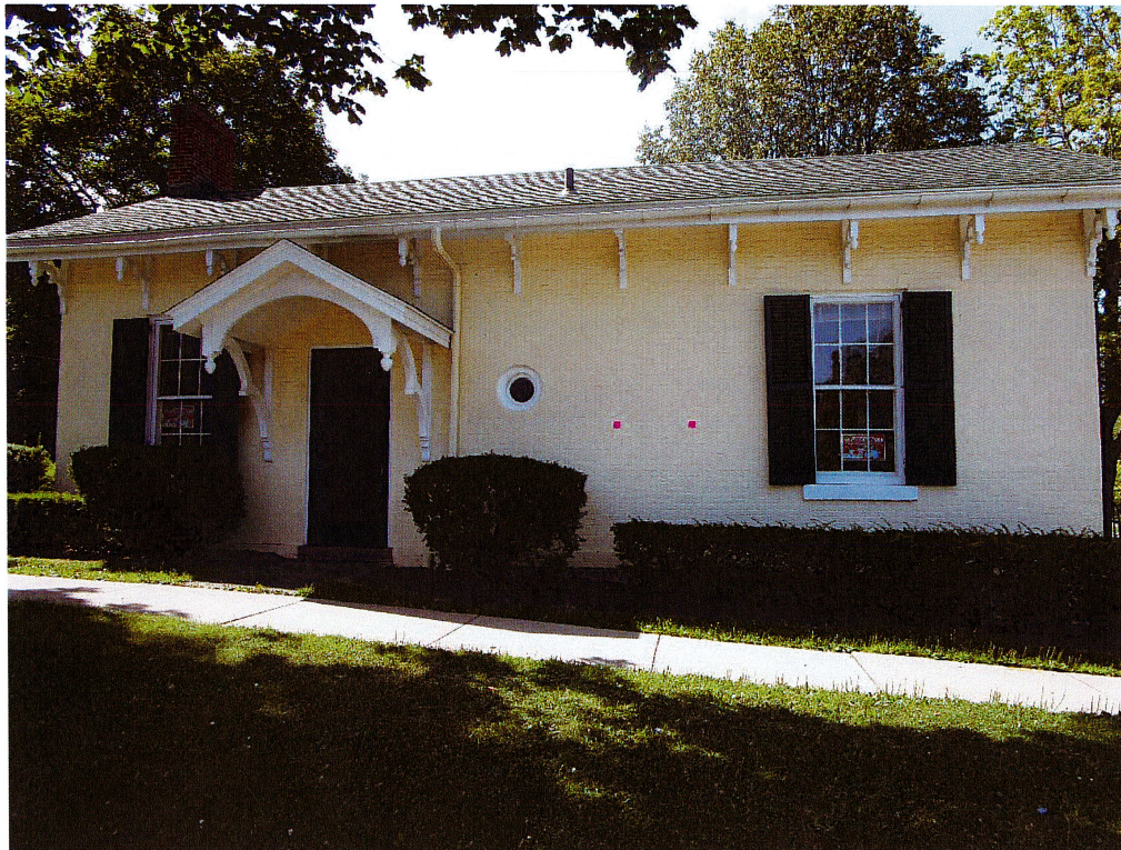
View from North Street looking south – view of secondary entrance. Dots are 36” apart.
