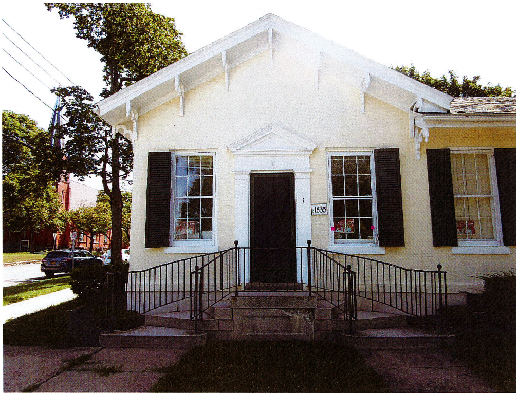
View of Main Street entrance. Dots on right window are 36" apart.
