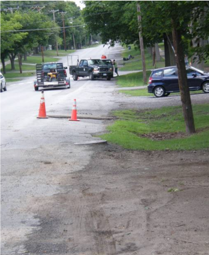
Figure 16. North Street's Current Condition (Source: Stuart I. Brown Associates)
