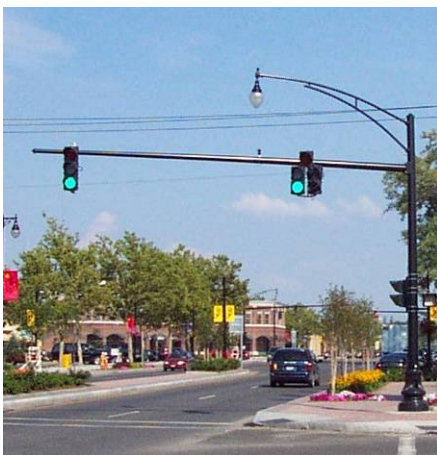
Figure 36. Example of a decorative signal pole (Source: Stuart I. Brown Associates)
